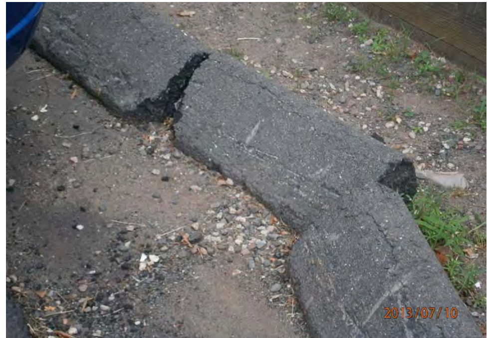
2. Asphalt curbing; damaged
