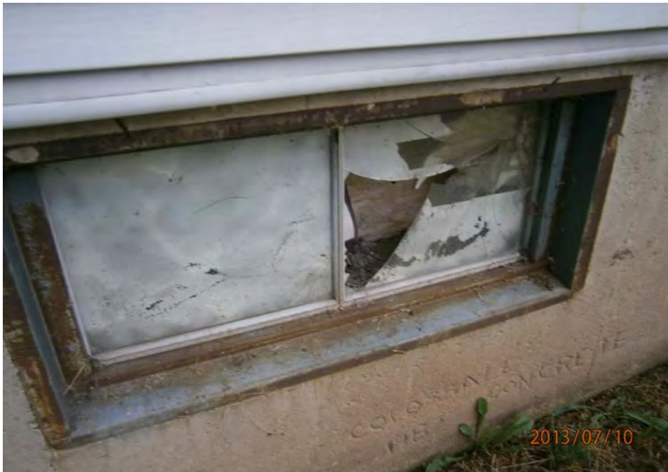
21. Basement hopper window; note broken glass
