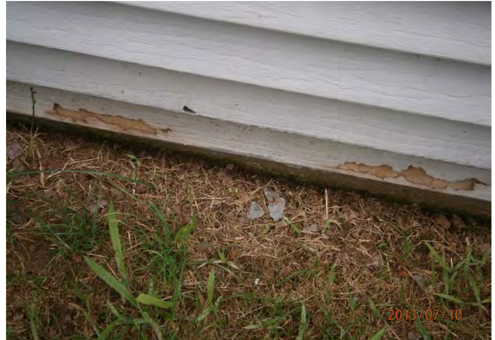
18. Siding; damaged
