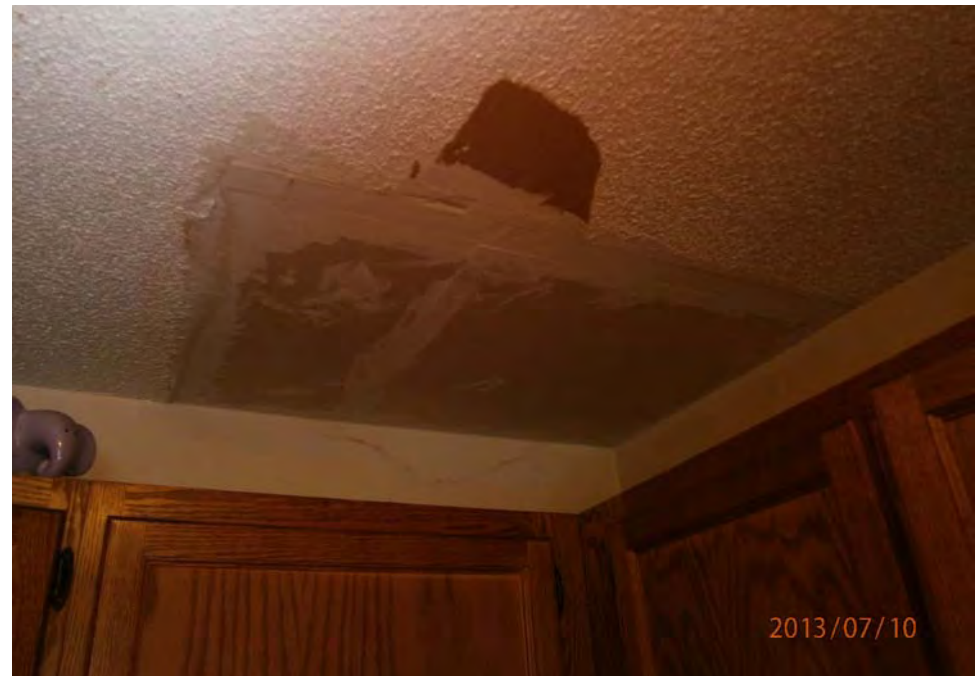
36. Unit ceiling moisture damage
