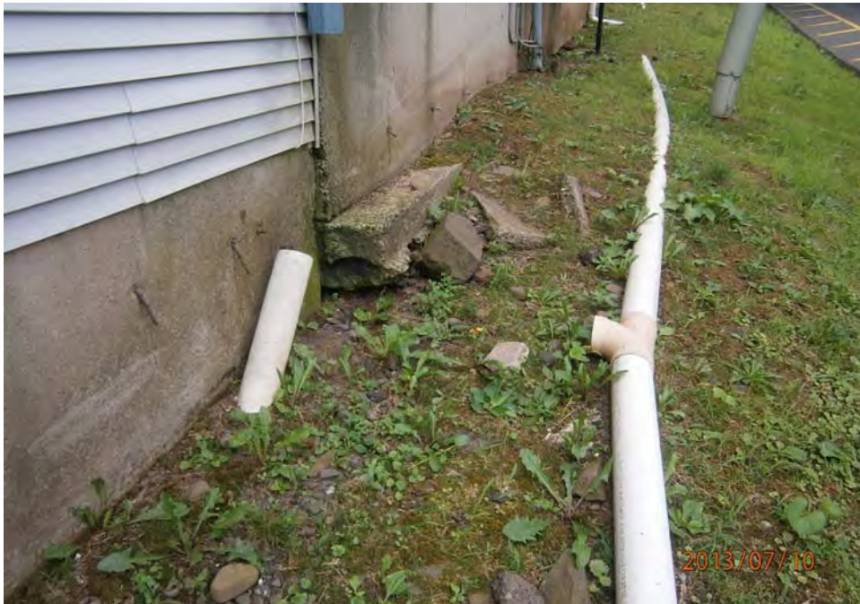
11. Storm drain lines; damaged
