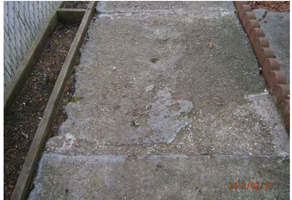
8. Concrete walkway; deteriorated
