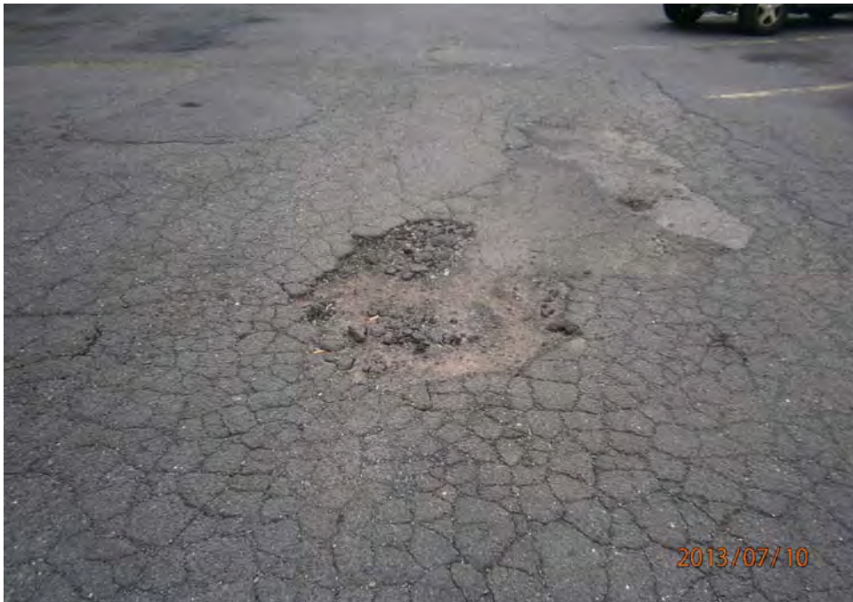
1. Asphalt parking area with potholes
