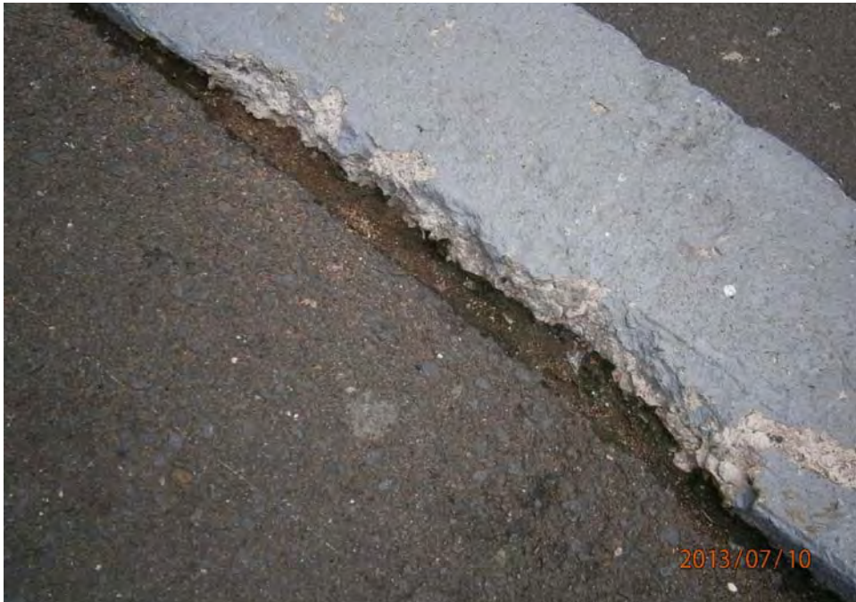
7. Concrete retaining wall needs repair
