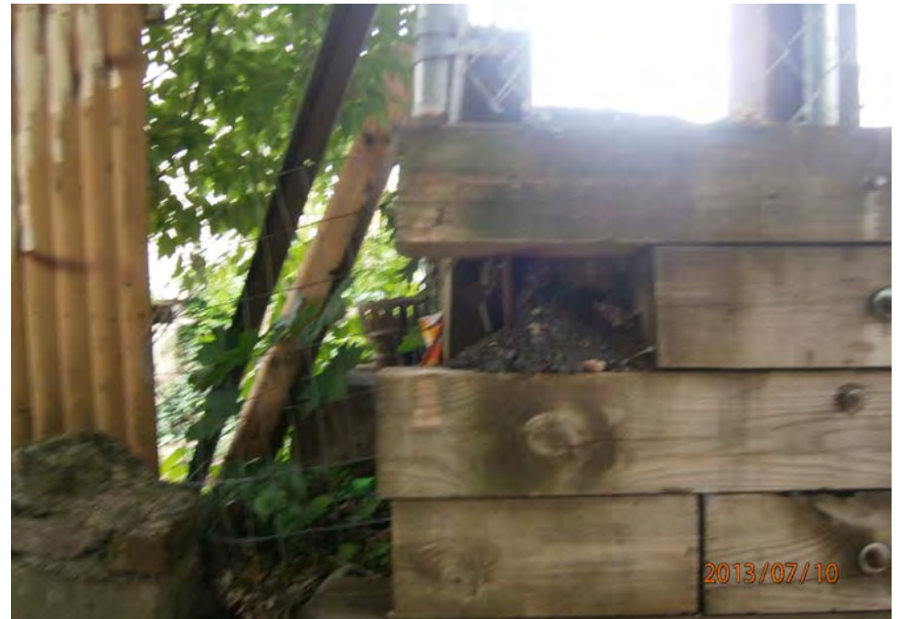
6. Minor damage to wood retaining wall
